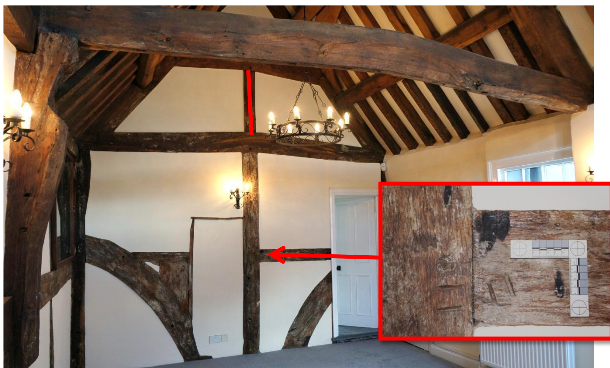
Figure 24 the front side of the rear range with its king post highlighted in red in the upper part of the image with evidence of the use of rush lights or "dip lights" to illuminate the room at mid rail height
