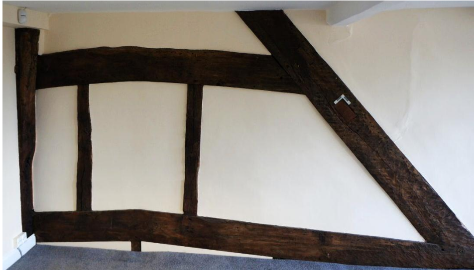
Figure 26 a queen post roof with cranked tie-beam belonging to 62 Fore Street exists at right angles (and therefore parallel to Fore Street) to a wall post of 63 Fore Street
