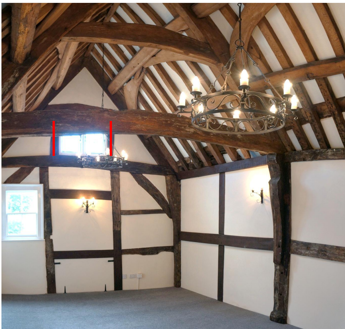
Figure 22 the rear 2 bay range of 63 Fore Street with its exposed timber frame with queen struts (in red) at the rear of the room and a central tie beam supported by gun-stock jowls
