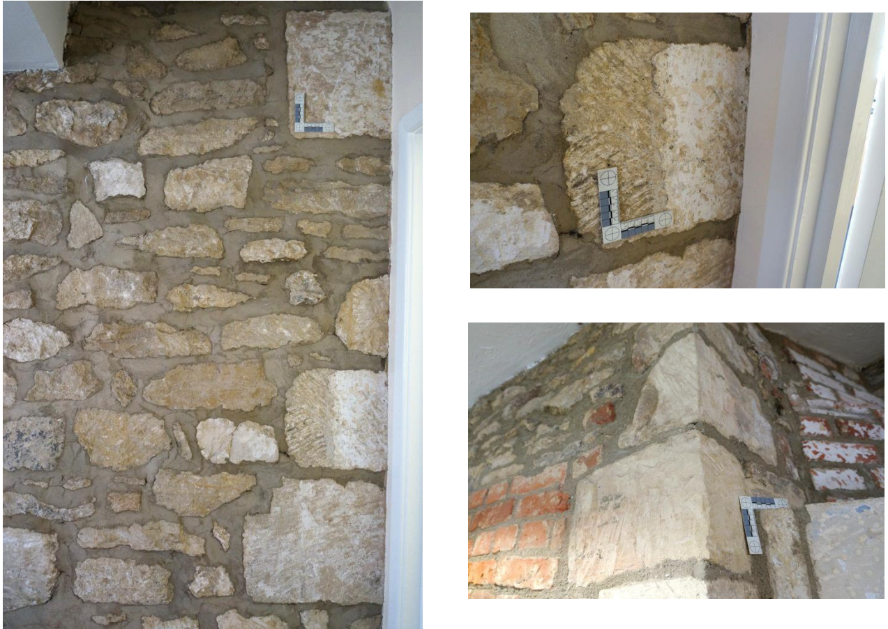
Figure 5 Re-used Limestone for quoins amongst the darker local stone (63 Fore Street)
