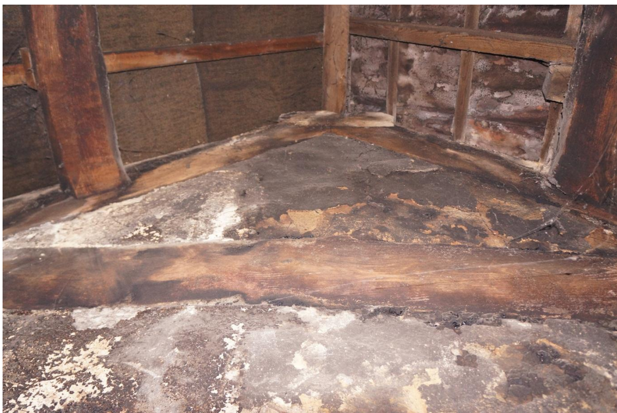
Figure 17 Evidence of heavy sooting and fatty crystalline deposits within the roof space above the hall of 9 Church Street
