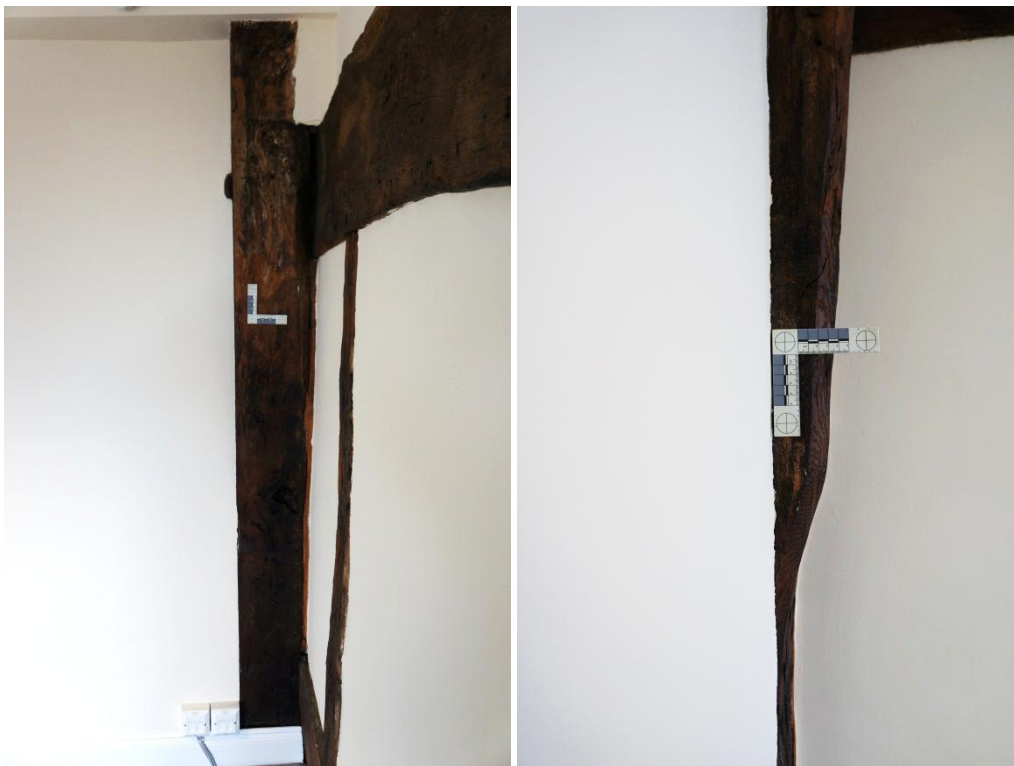
Figure 25 a corner wall post above the main body of 3 Fore Street suggesting a separate timber frame from that of the coeval solar behind it
