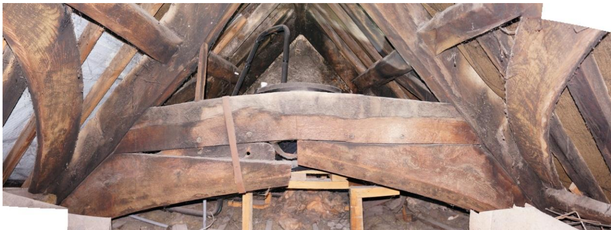
Figure 14 the arch-braced and cranked collar above the once open hall at 9 Church Street
