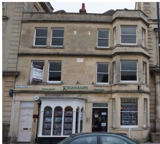
Figure 19 the 1789 stone clad front of 63 Fore Street, Trowbridge. This Georgian facade masks the original timber-framed structure and uses a raised parapet to obscure the two roof gables
