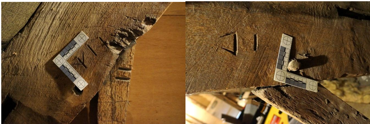
Figure 29 carpenters marks found in the reused timbers of the main roof of 63 Fore Street
