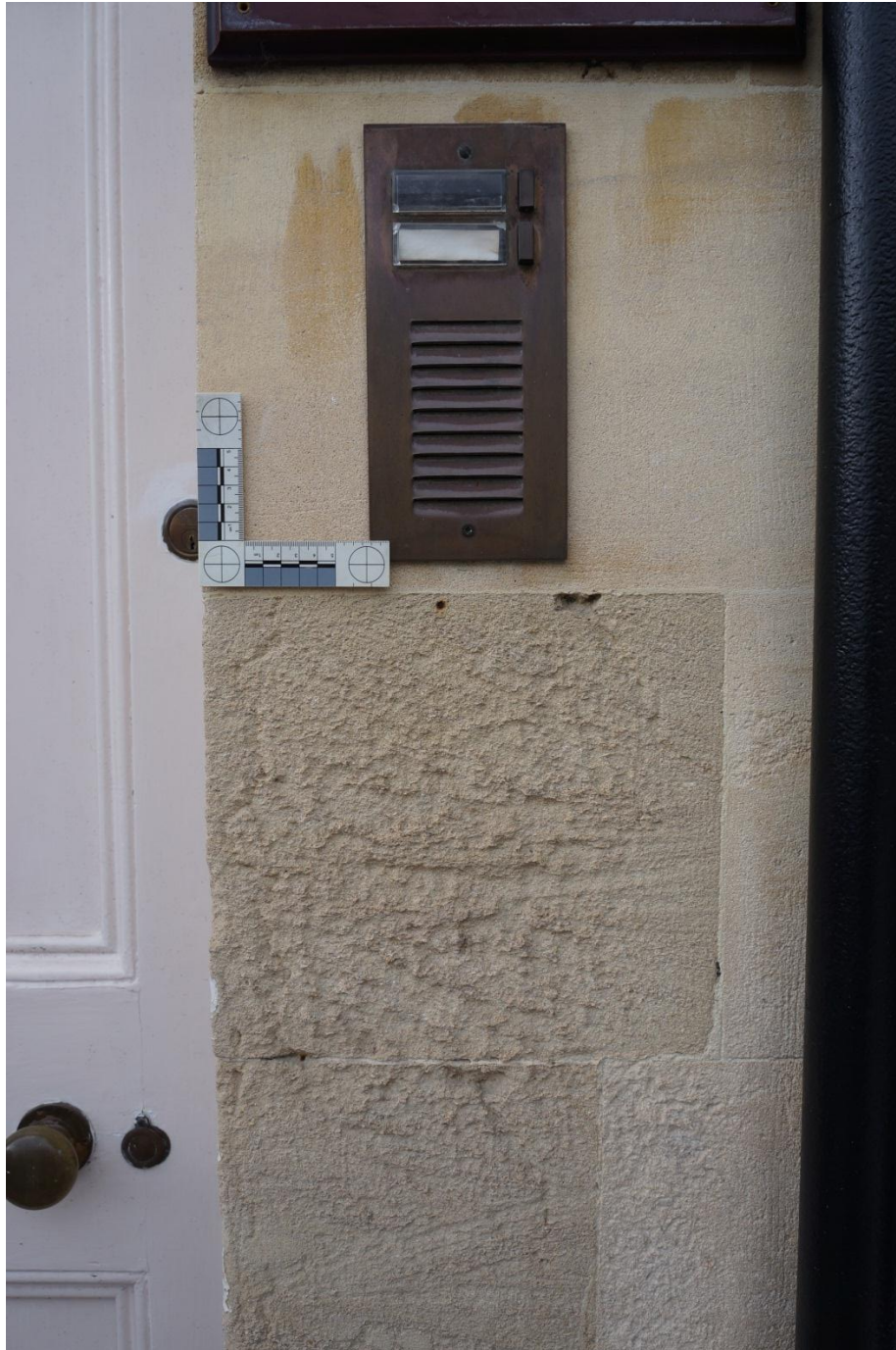
Figure 6 Georgian stone cladding c1789, used to re-front the medieval core of 63 Fore Street
