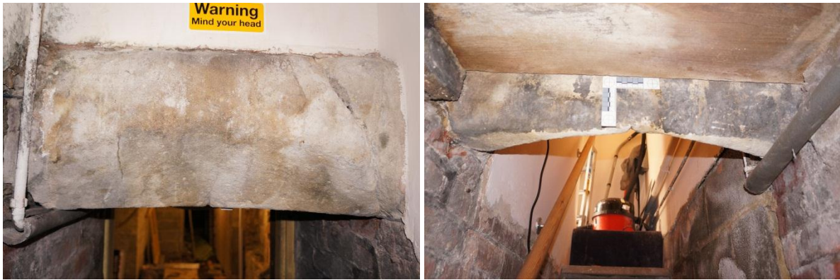
Figure 11 a well-shaped and re-used stone lintel above the entrance to the undercroft of 7 Fore Street, Trowbridge
