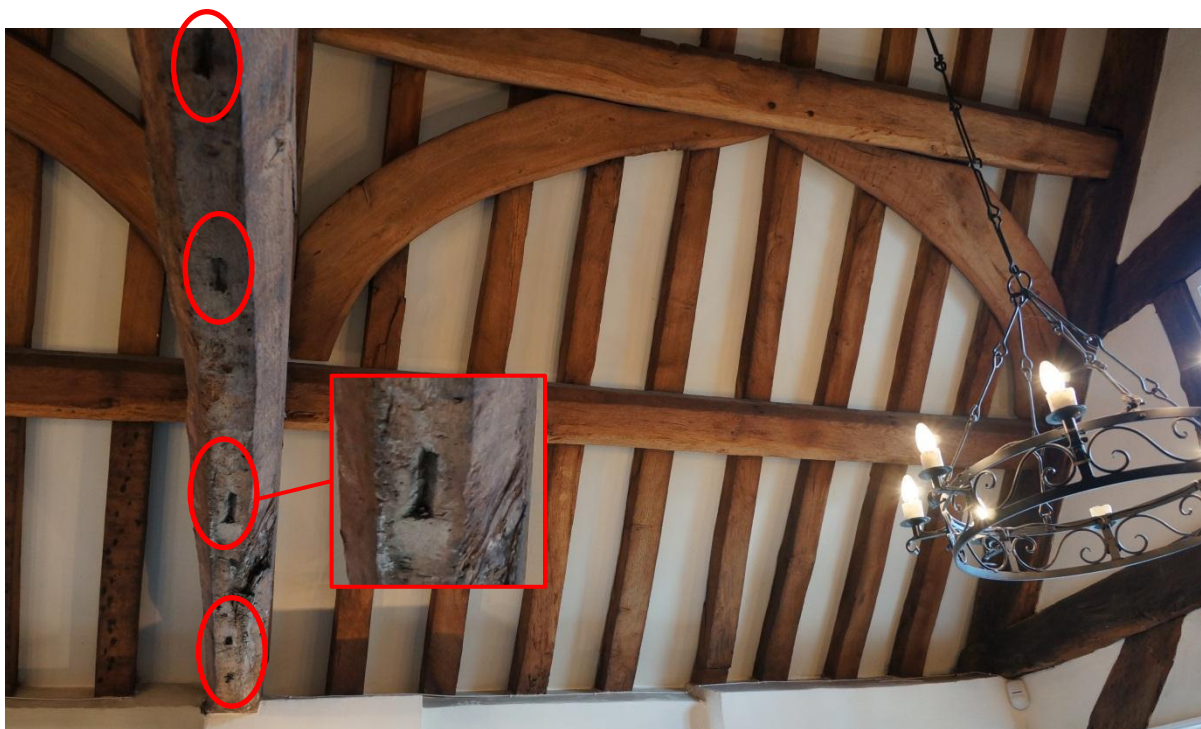
Figure 23 evidence of shallow mortises cut sometime after the initial construction to house a partition to separate the open two bays into two rooms
