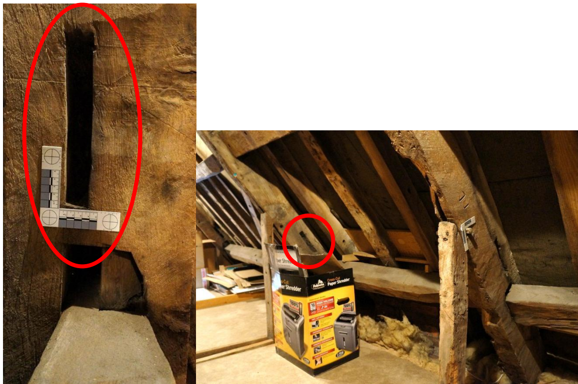
Figure 20 re-used roof timbers above 63 Fore Street with empty mortises highlighted
