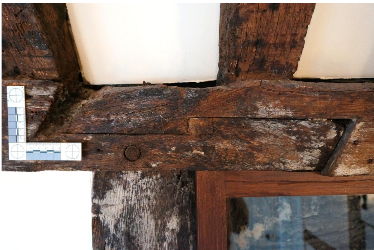
Figure 32 a previously unseen undersquinted butt in a halved and tabled scarf with key in the Solar of 63 Fore Street
