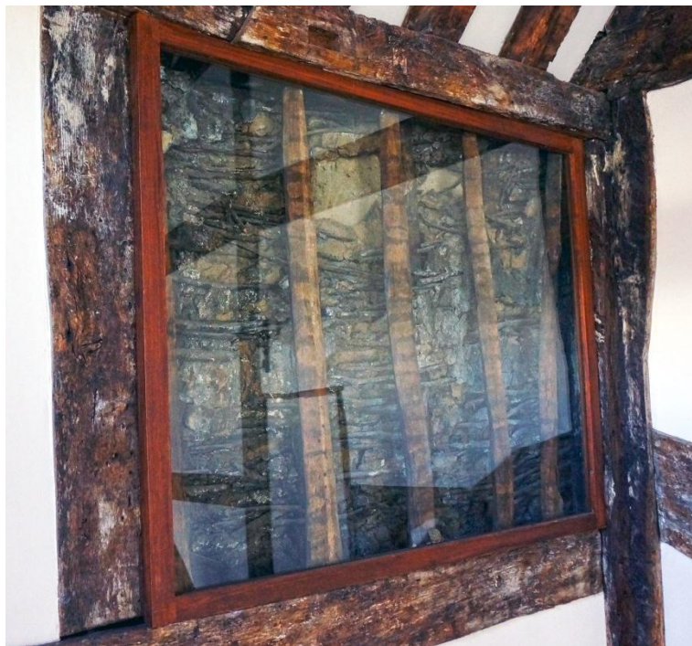
Figure 27 the wattle and daub from the solar wall has been removed to expose the wattle and daub of 62 Fore Street. The timber staves (uprights) belong to the solar
