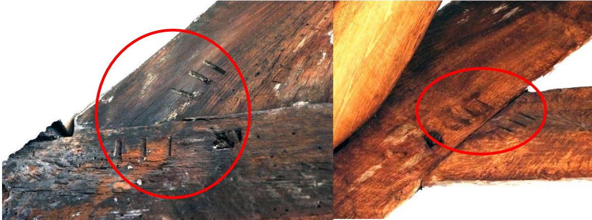
Figure 28 carpenters marks found in the Solar of 63 Fore Street
