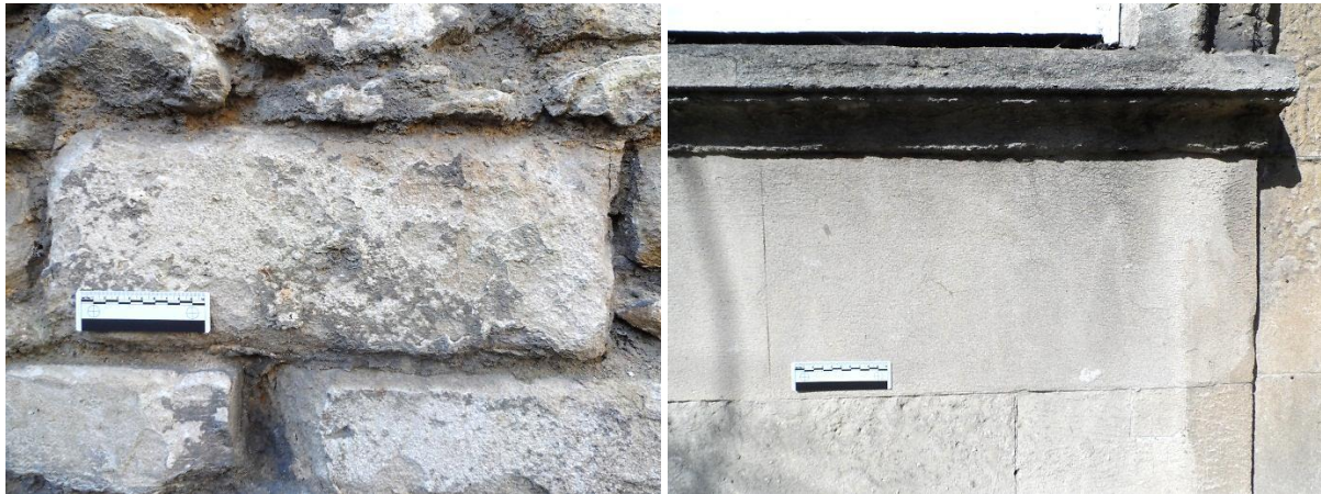
Figure 3 An example of re-used Oolitic Limestone (most likely from Dorset) in the walls around Trowbridge - above left - and the yellower local sand stone used in later Georgian fronts - above right
