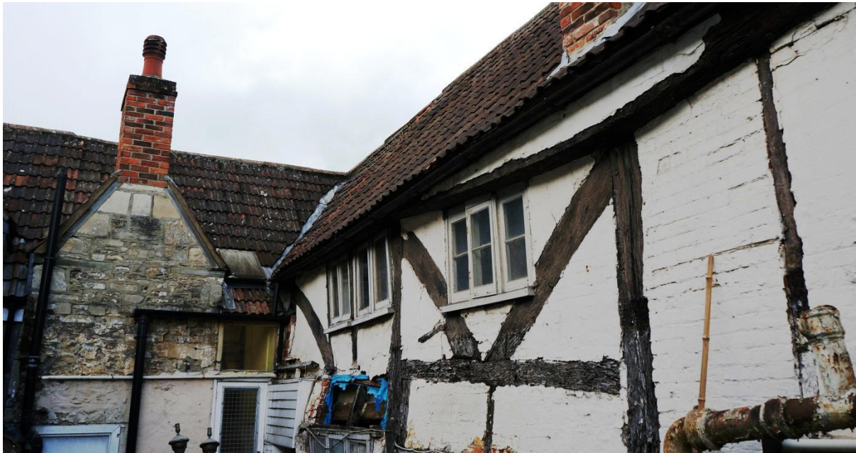
Figure 16 the rear of 9 Church Street showing a chimney on the rear wall of the hall and the later added wing on the right of the picture
