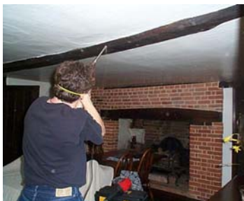
Photo 3: Extraction of a core in progress
