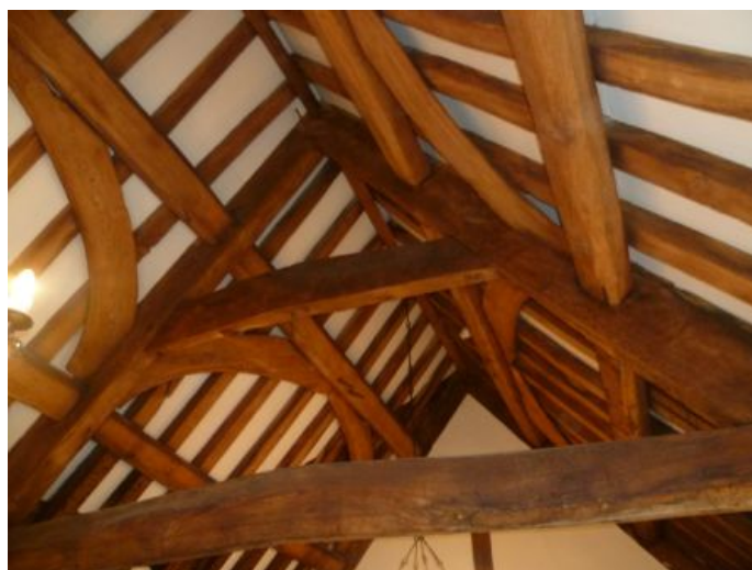
Photo 1: Roof truss of the rear range of 63 Fore Street
