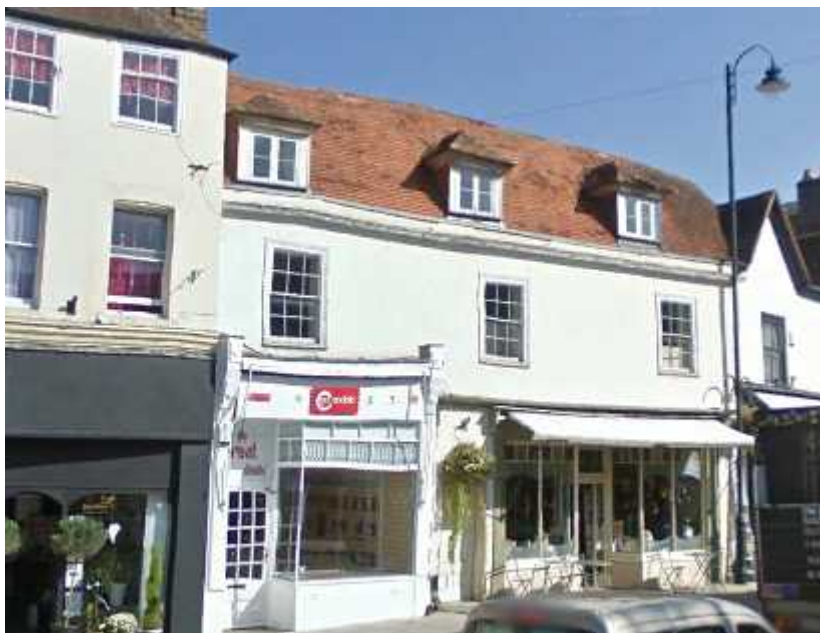
Photo 1: 6 High Street – south aspect
