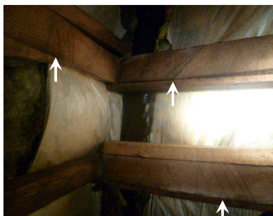
Photo 8: Carpenter's marks at the apex of rafters
